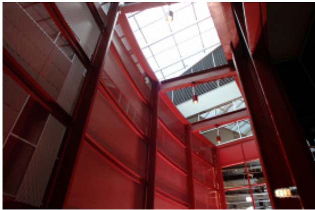
Reginald F. Lewis Museum, Stair Volume The atrium skylight provides dramatic illumination for the central stairs. Photograph by Carl Caruso
