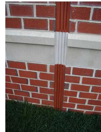
PVC Expansion Joint Cover
