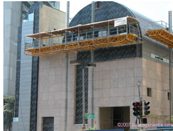
Insulation and Finish Masonry at Exterior
