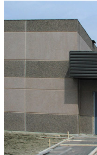
PVC Expansion Joint Cover
