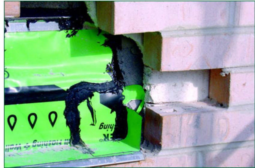
In Real Life (At flashing termination)
