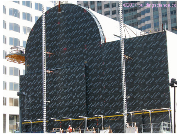
Self-applied Air Barrier
