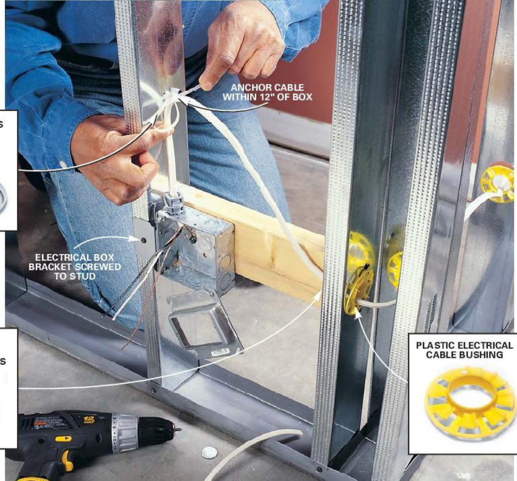
PLASTIC TIE SECURES ELECTRICAL CABLE
