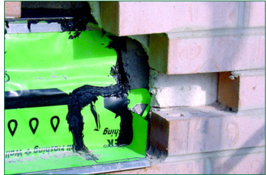
In Real Life (At flashing termination)
