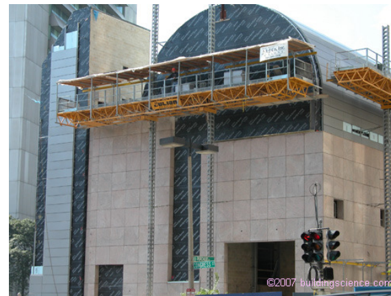
Insulation and Finish Masonry at Exterior
