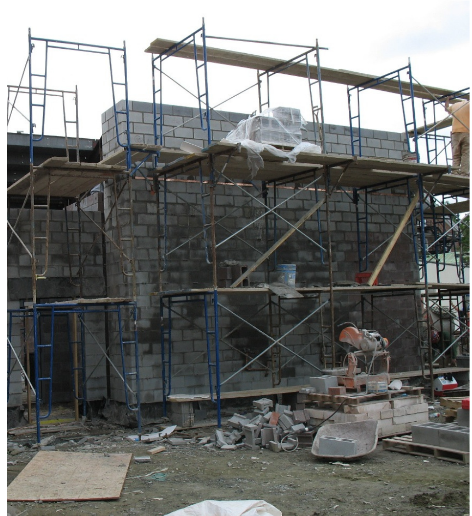
Fire-rated Masonry Enclosure
