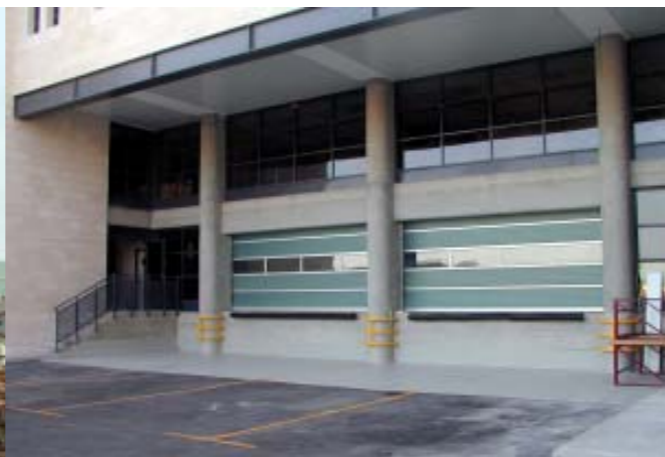
Loading Dock West Elevation
