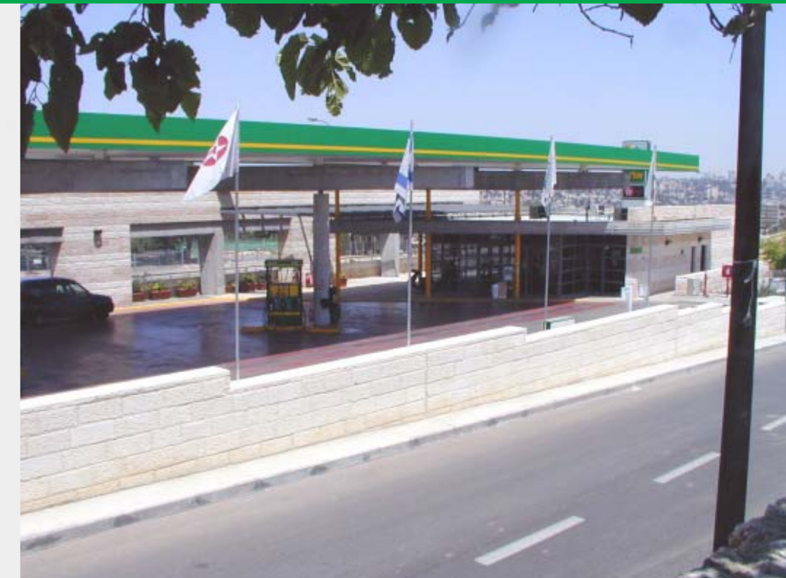
Construction Phase, View towards Bethlehem
